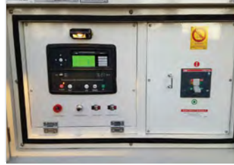
REAR CONTROL PANEL WITH MLCB
