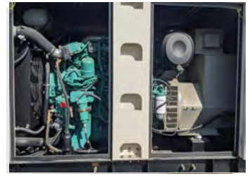
EASY ACCESS FOR MAINTENANCE
